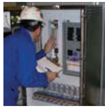
Control and Monitoring
